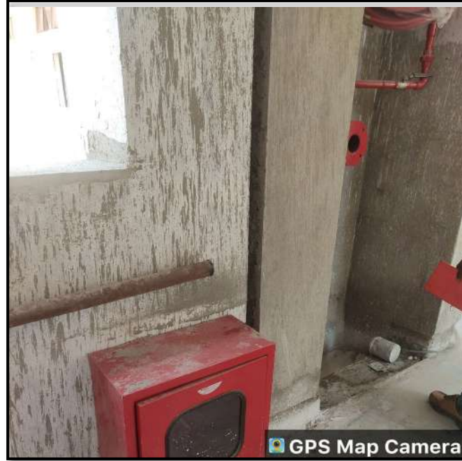
Obstruction in passage due to Hose Reel Cabinet
