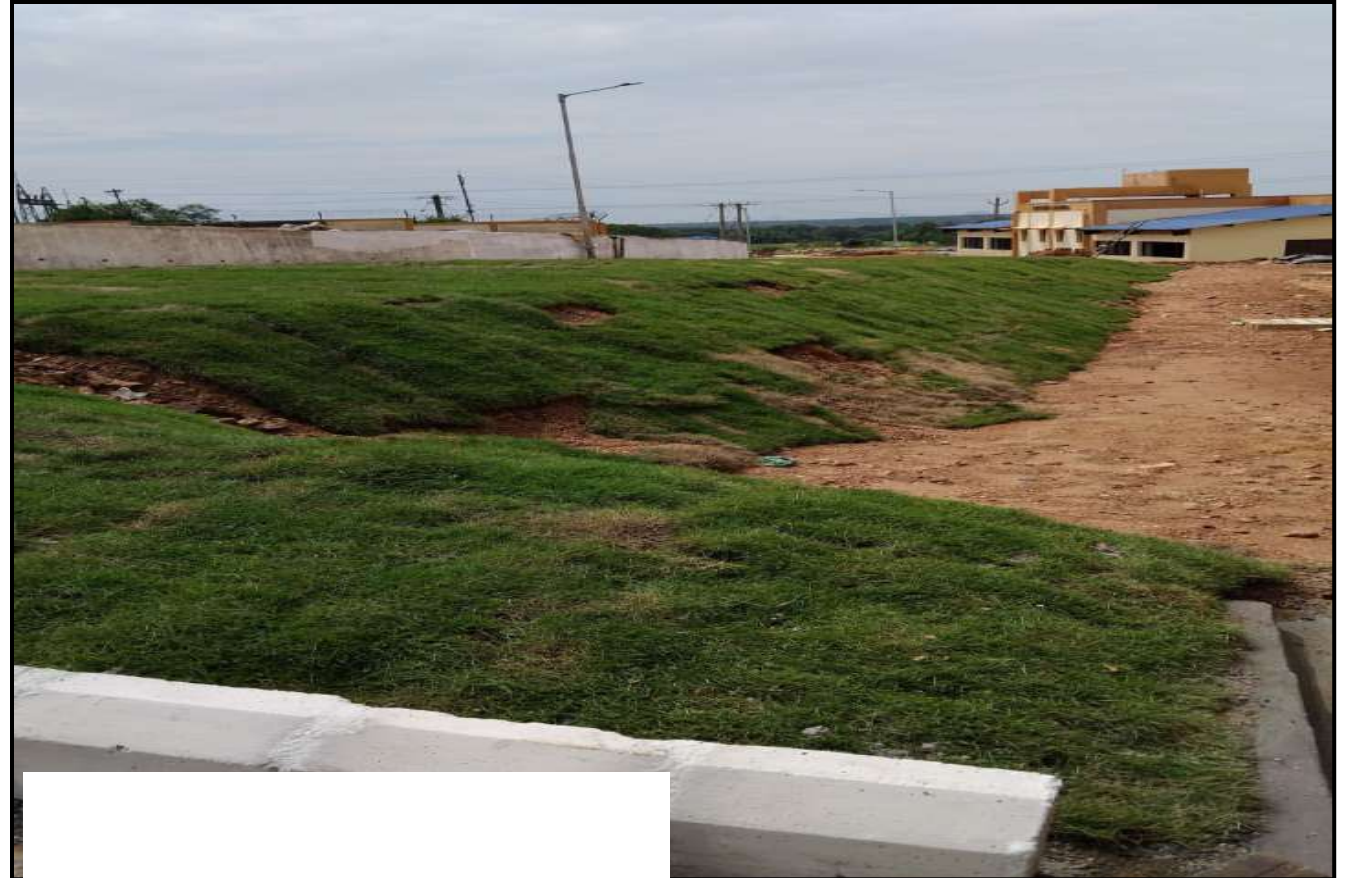
Vegetation/Landscaping used to retain the slope
