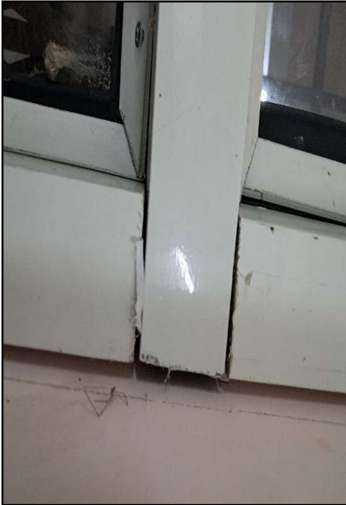
Aluminium door joints not mitred properly
