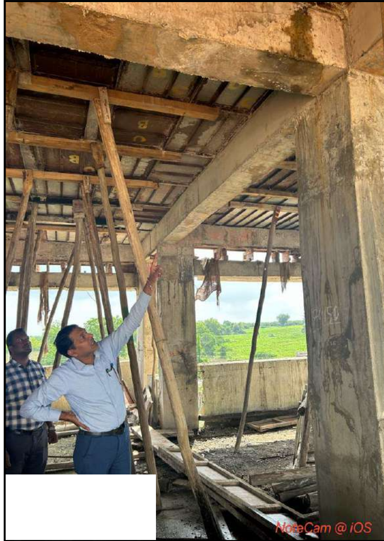
Leakage of slurry due to substandard Shuttering
