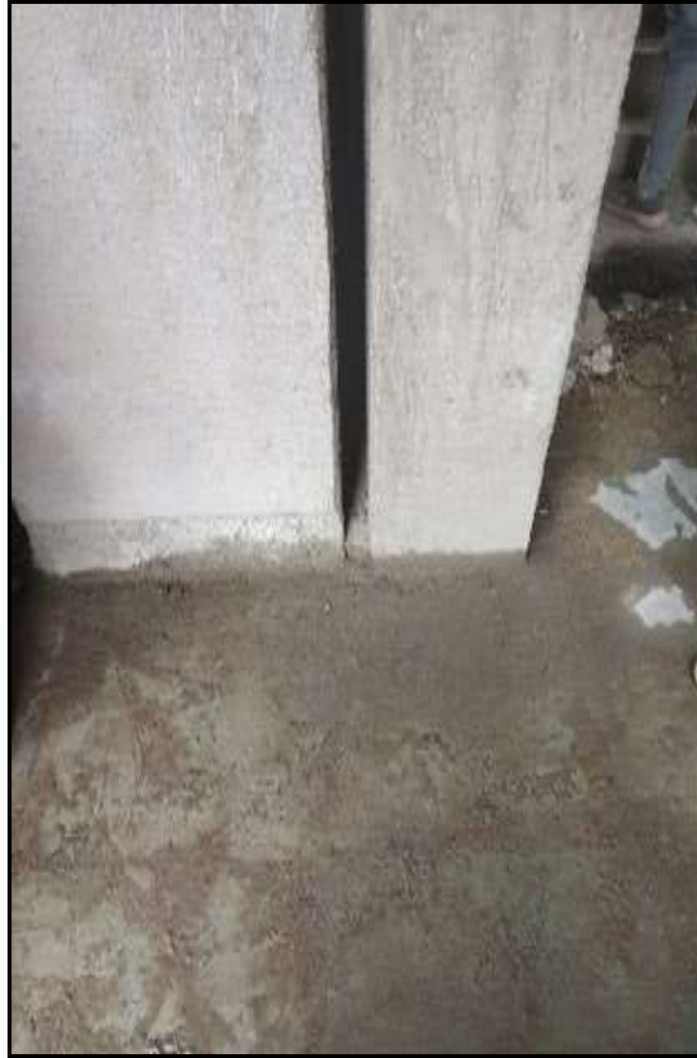
Flooring done over the expansion joint
