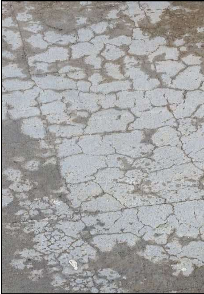
Cracks in waterproofing
