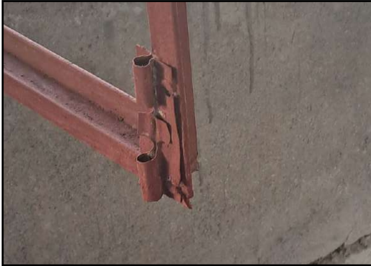
Joints not flush welded
