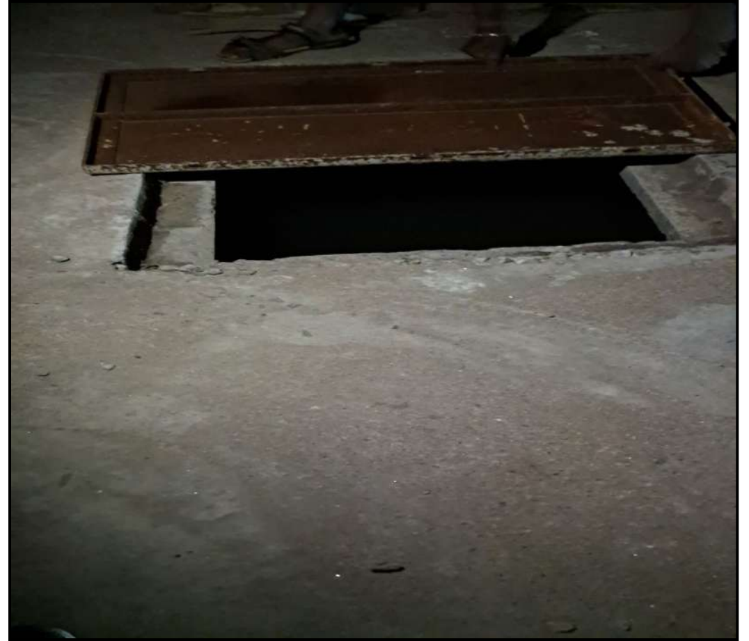
Water Tank cover not proper
