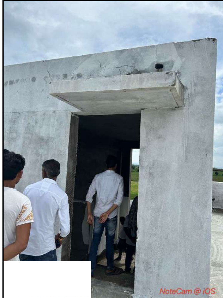
Mismatch in door opening & Projection
