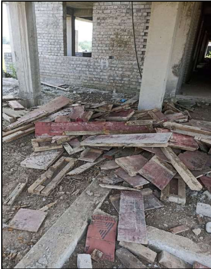
RCC with poor shuttering
