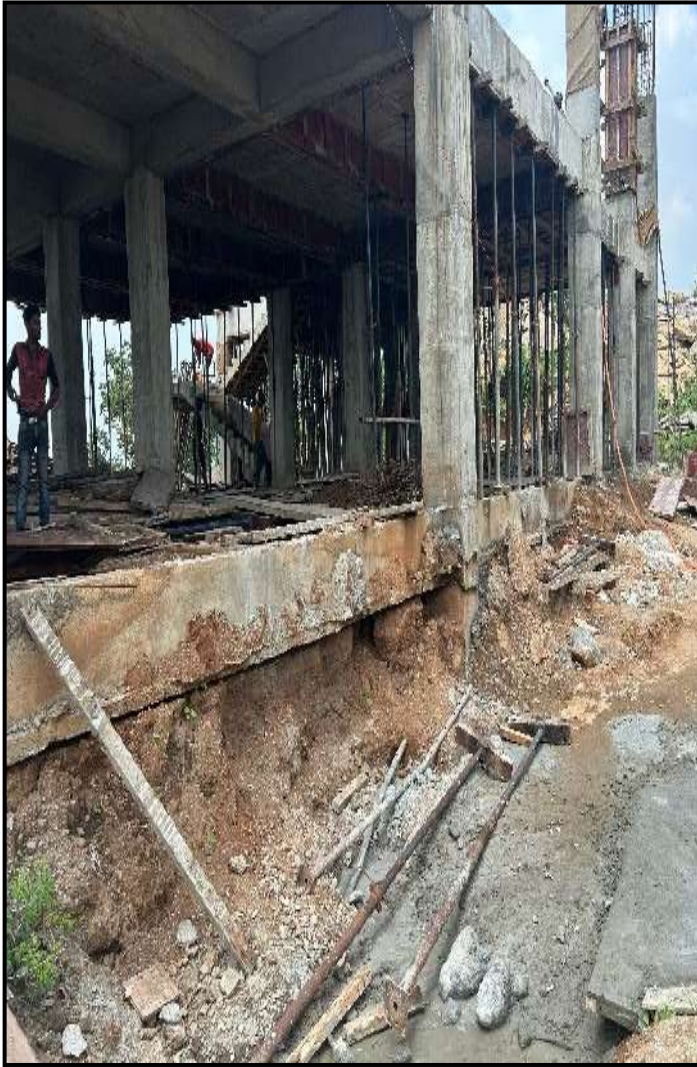
No brickwork below plinth beam
