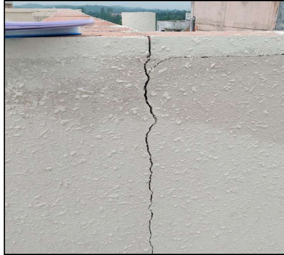
Cracks in Parapet Wall
