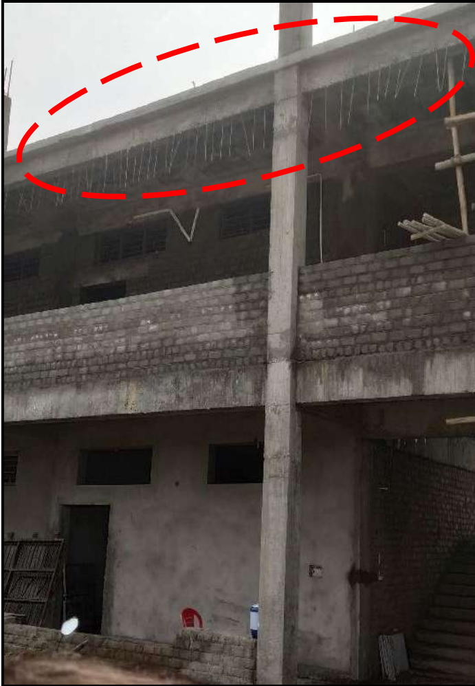
Casting of fins not made integrally with beam
