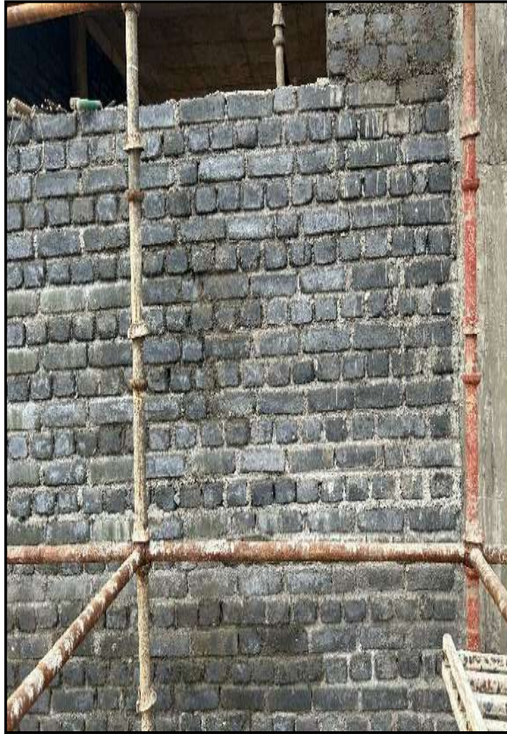
Joints not filled properly
