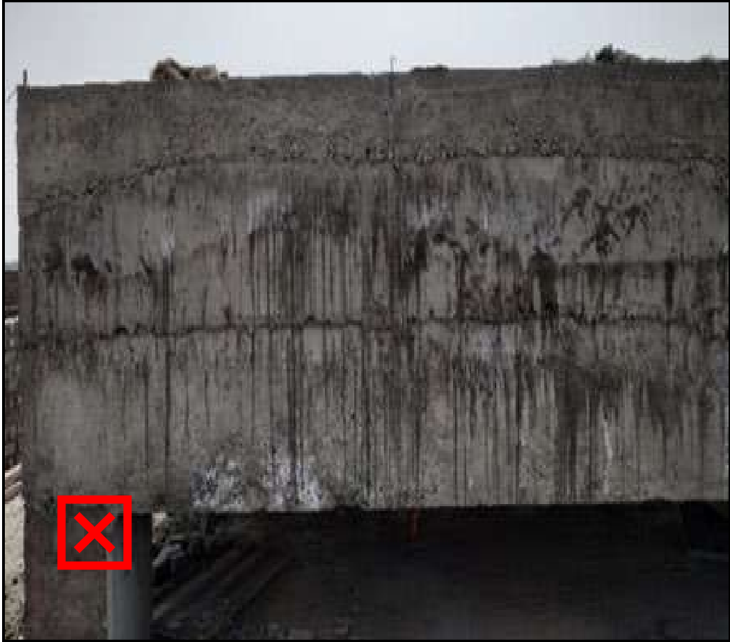
OH Tank wall casting not continuous
