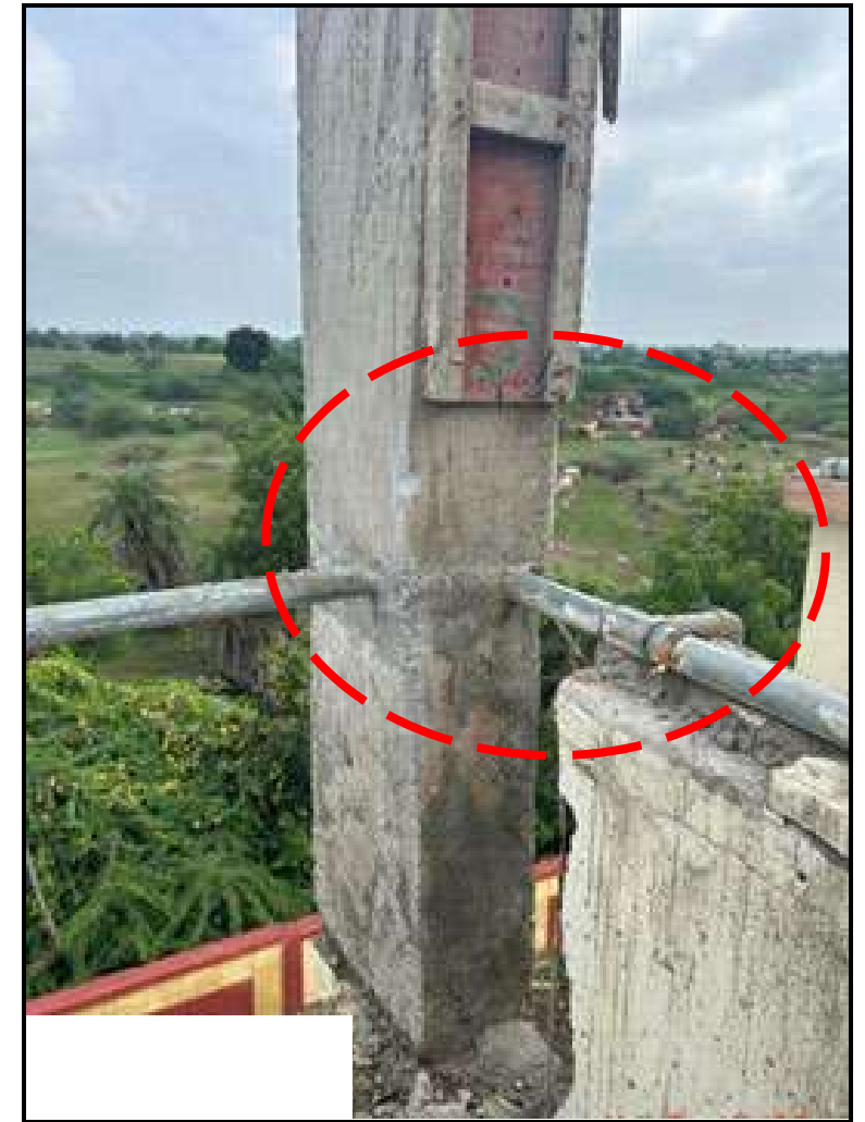
Water pipeline casted in column
