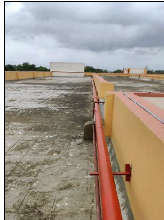
Fire Pipe installation is supported by clamps at Parapet Wall
