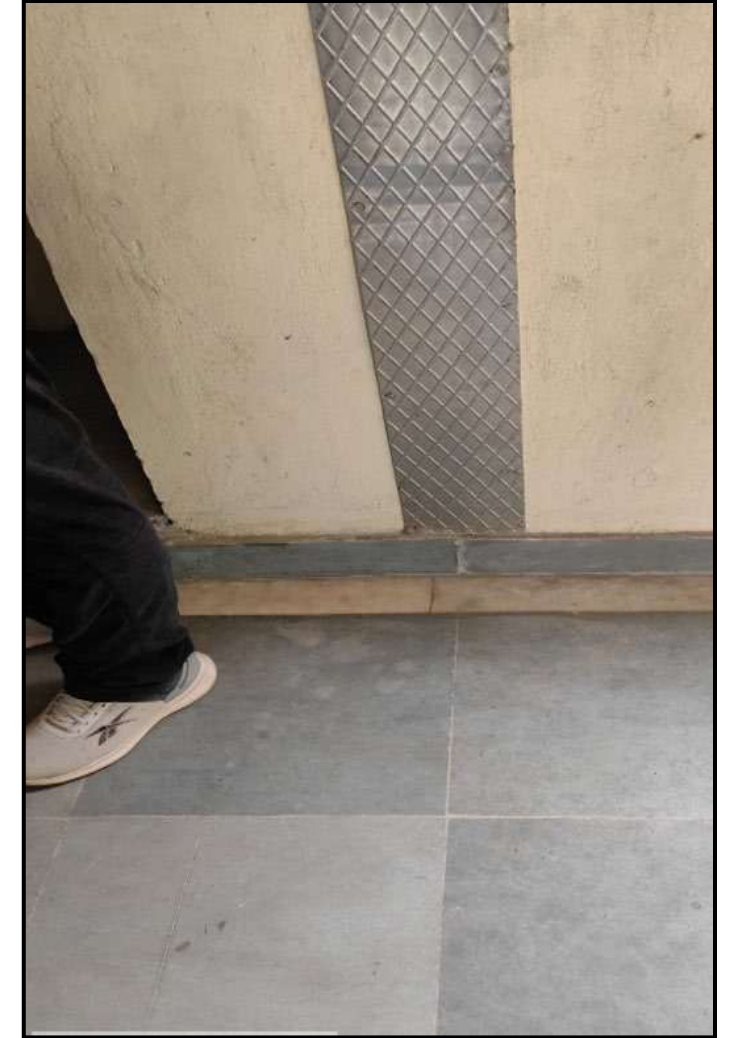
Expansion Joint missing in floor
