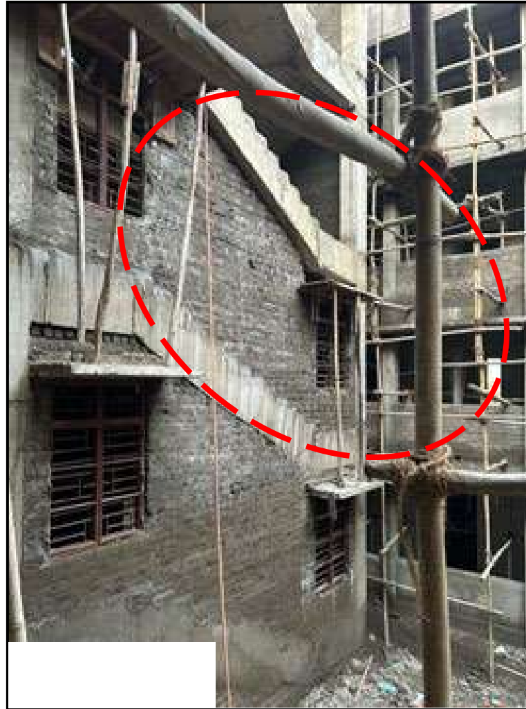
Stair flights not symmetrical
