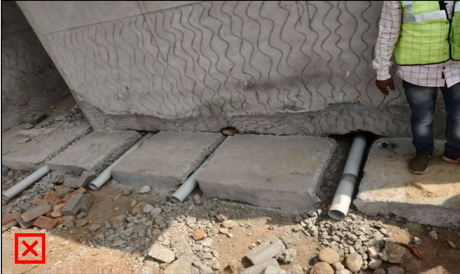
Bad work: Plinth Protection Damaged
