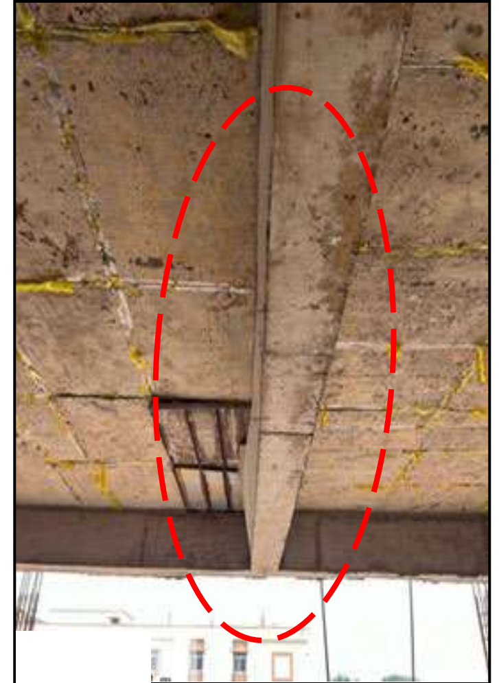
Beam is not in alignment
