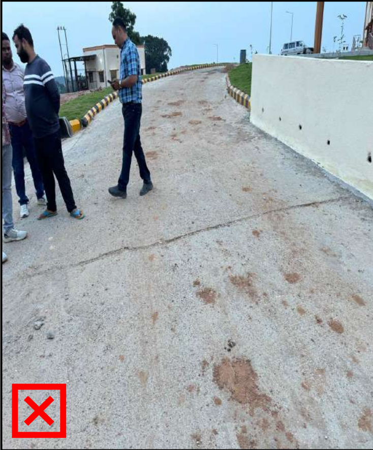
Road Expansion Joints not proper
