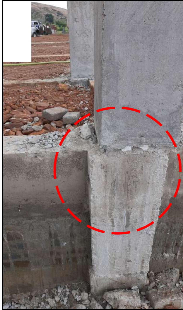
Zig Zag Column - Twisted bar
