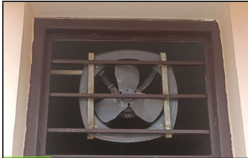
Improper Ex. Fan Installation
