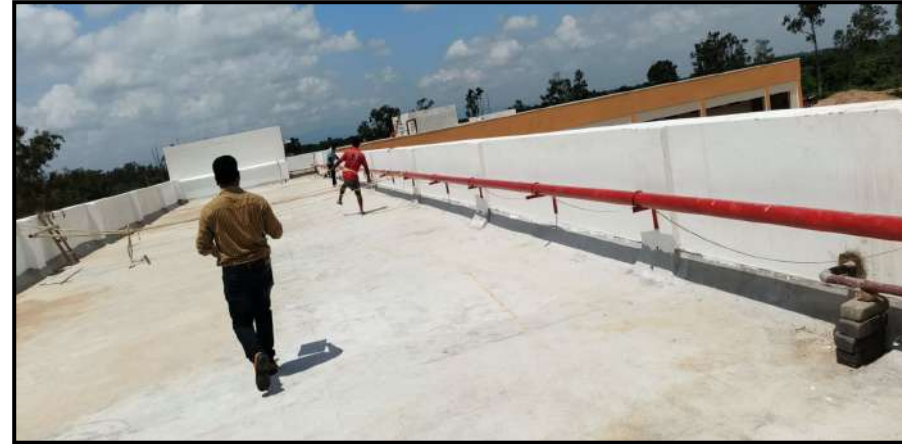
Fire Pipe installation is supported by clamps at Parapet Wall
