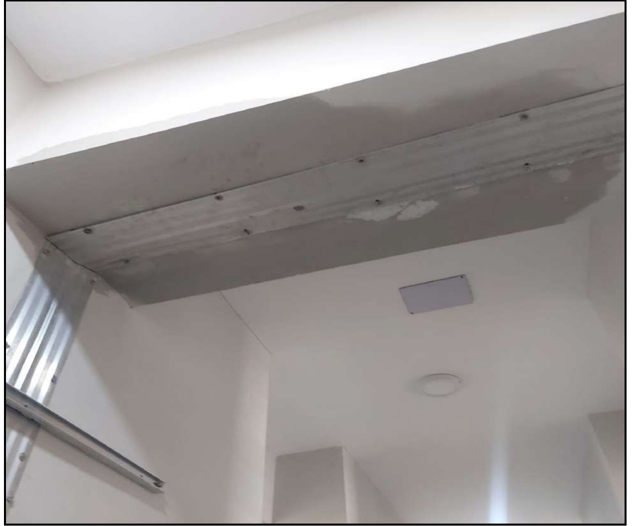
Dampness near expansion joint
