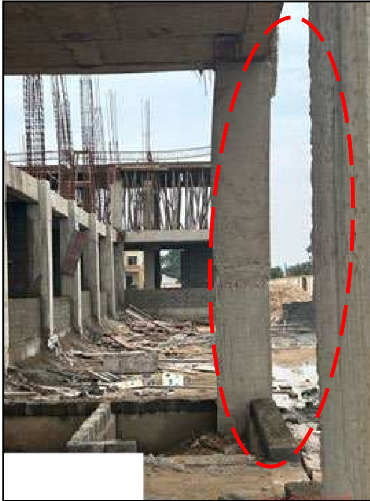
Column is not in alignment
