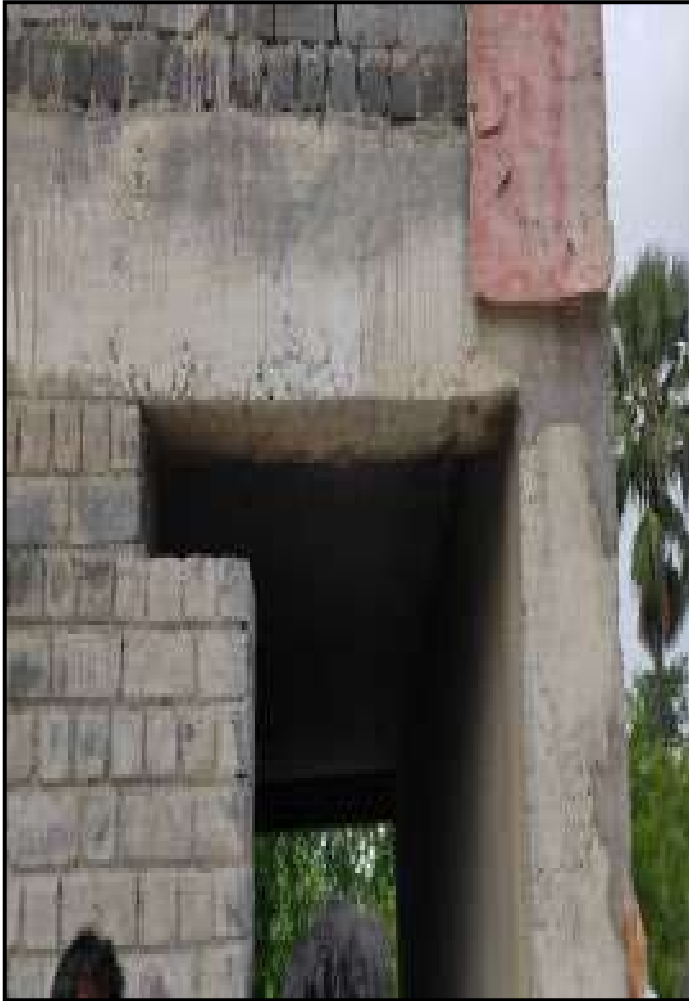
Column is to be cut for lintel
