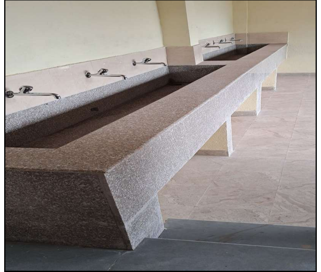
Trough: At least 2 nos waste holes required in trough
