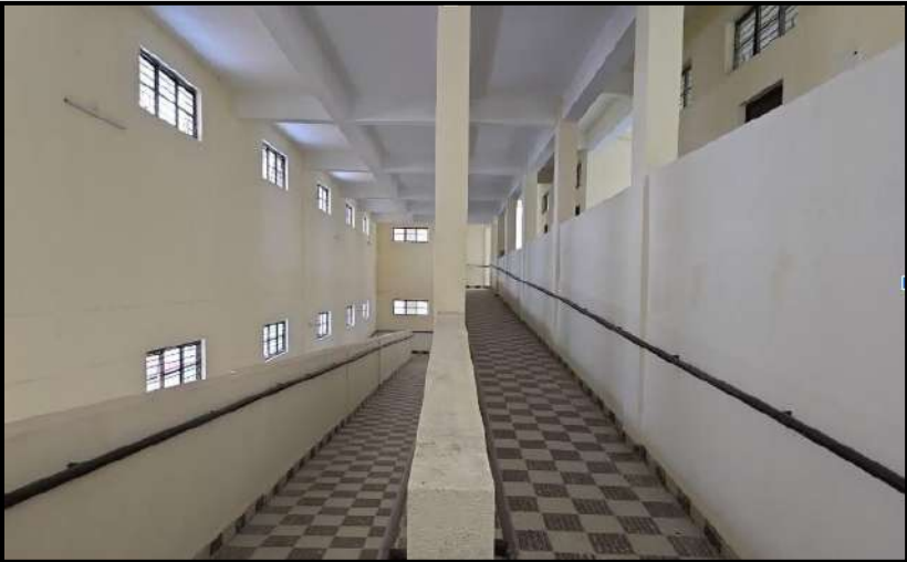
Antiskid & Tactile flooring in ramps Missing
