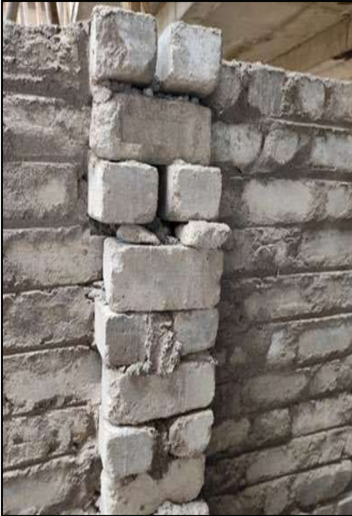
Joints not filled with mortar
