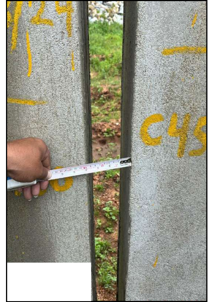
Expansion joint > 50 mm
