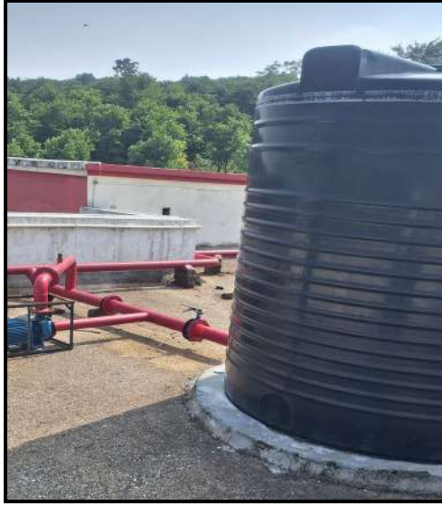
Wrong Placement of Fire Tank at Terrace
