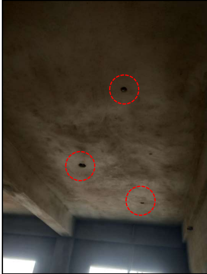
Improper Alignment during Slab Casting
