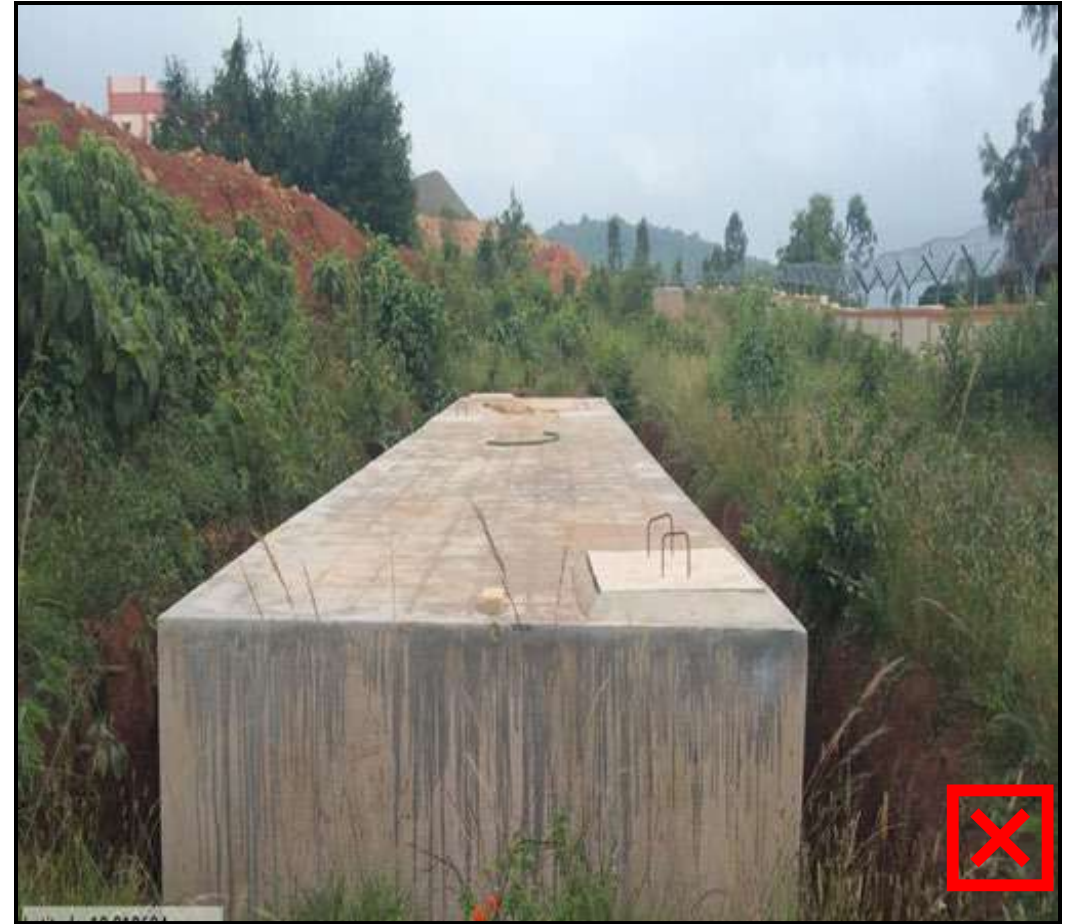
Bad work: Inlet/outlet chamber missing
