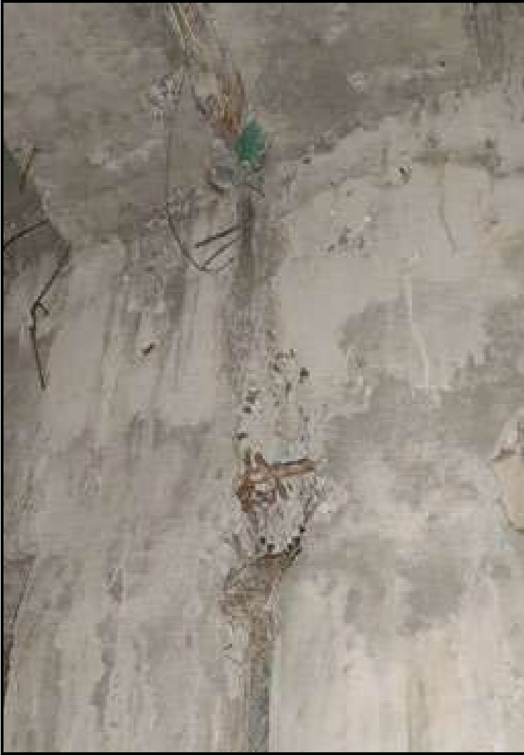
Beam casted continuous on expansion joint
