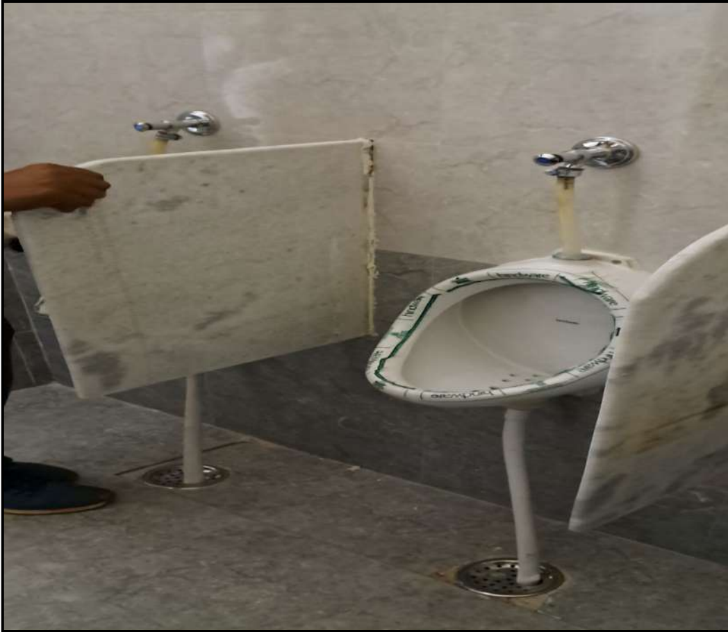
Urinal Partition & Floor trap not proper
