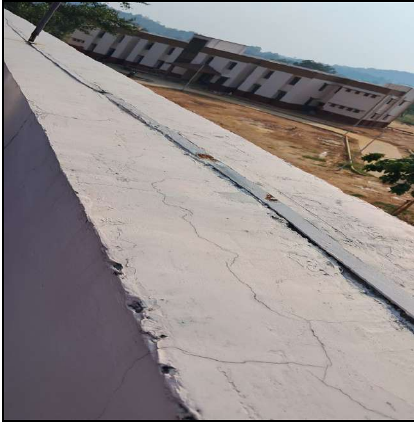
Cracks in coping
