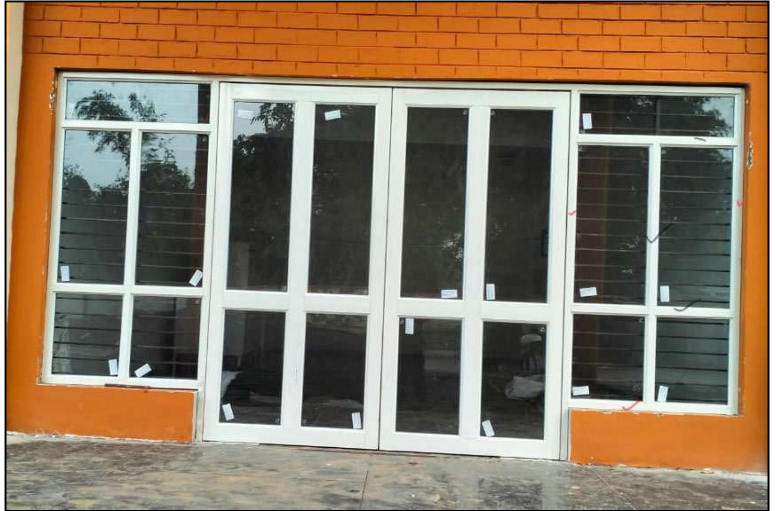
Correct way of fixing aluminium door
