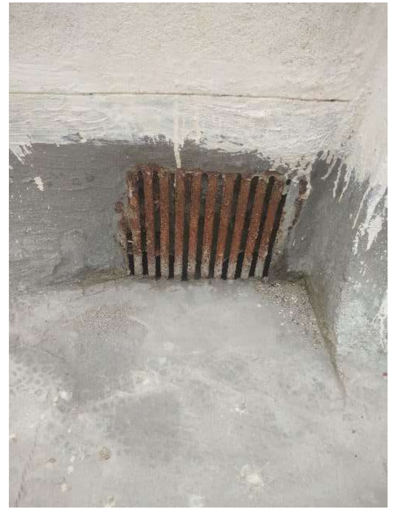
Grating is not as per specification
