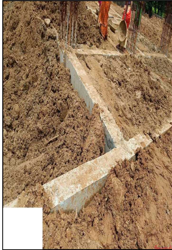
Backfilling not compacted
