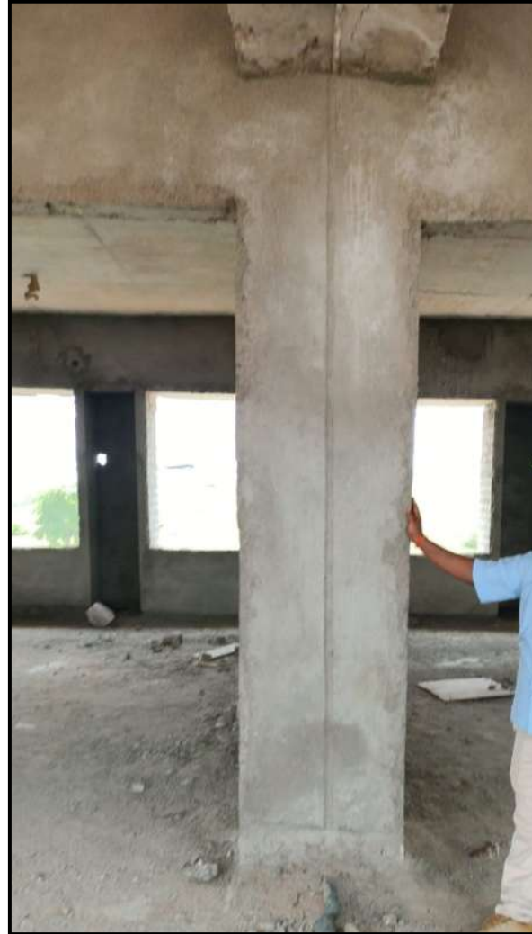
Expansion Joint filled with mortar
