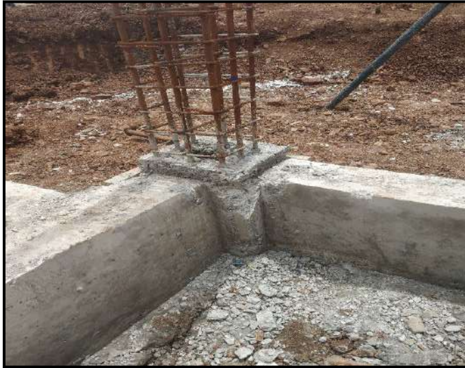
Poor Column Starter Quality
