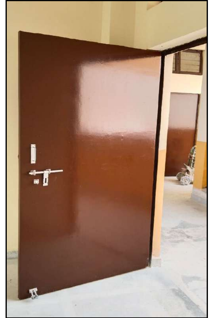
Correct way of fixing door fittings
