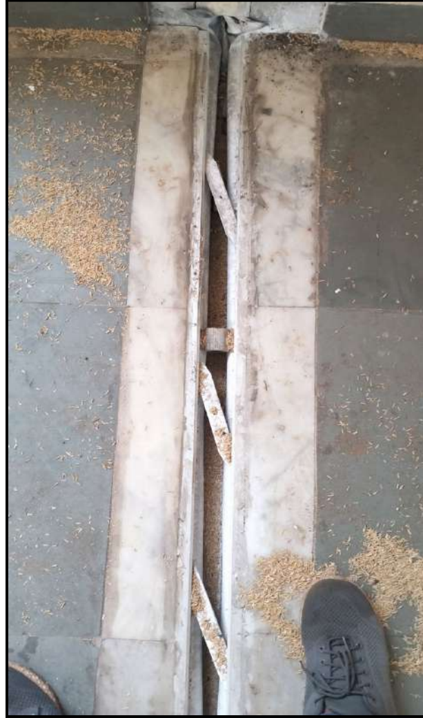
Expansion joint in floor
