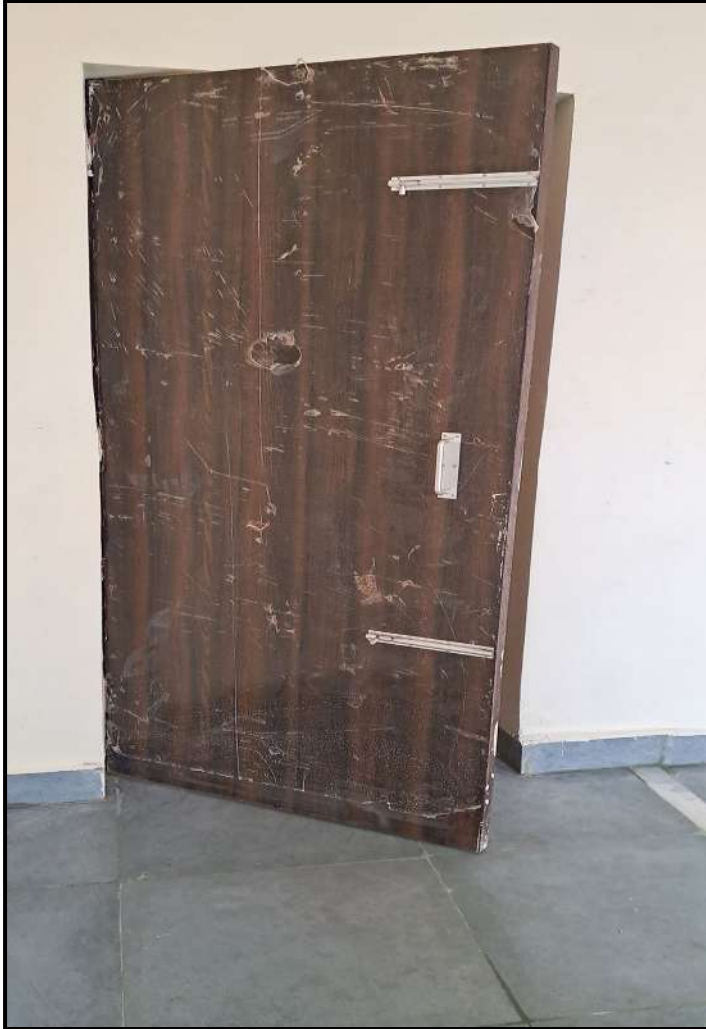
Tower Bolts: Fixing not proper
