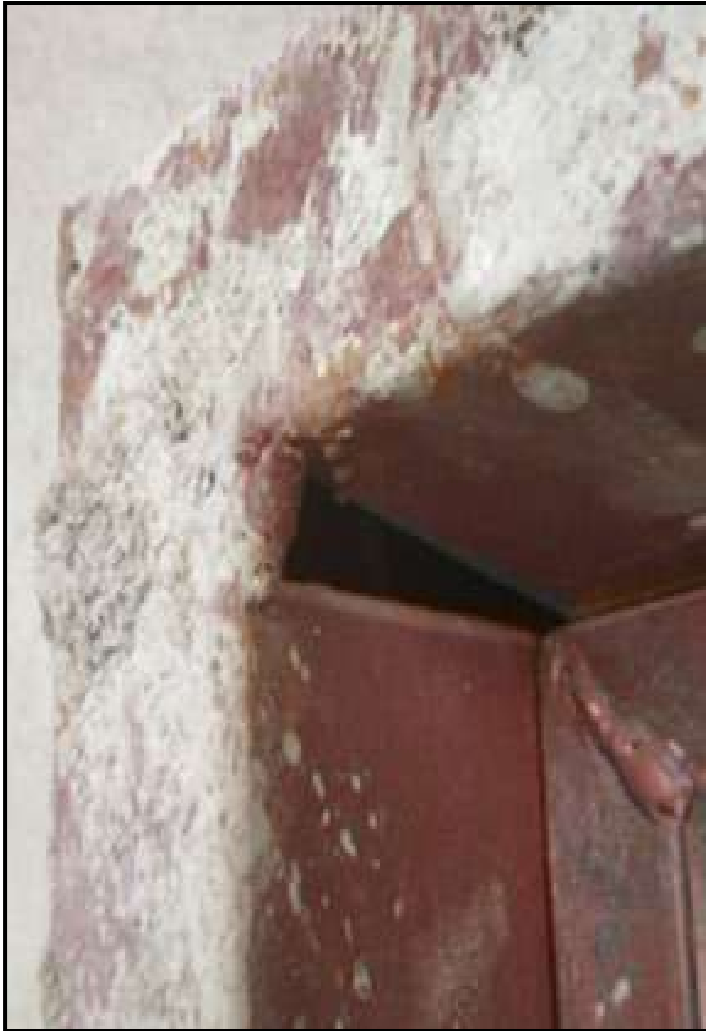
Window without flush butt welding
