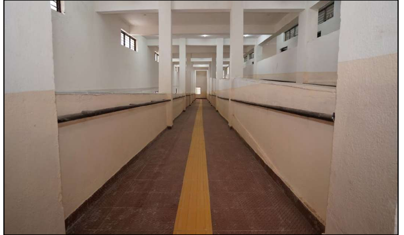
Tactile flooring in ramps Provided
