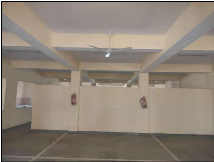
Wrong placement of Fire Extinguishers
