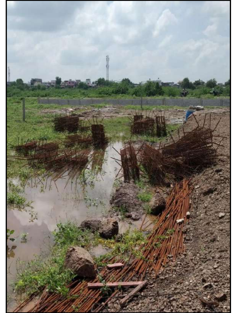
Stacking of Steel in Low Lying Area
