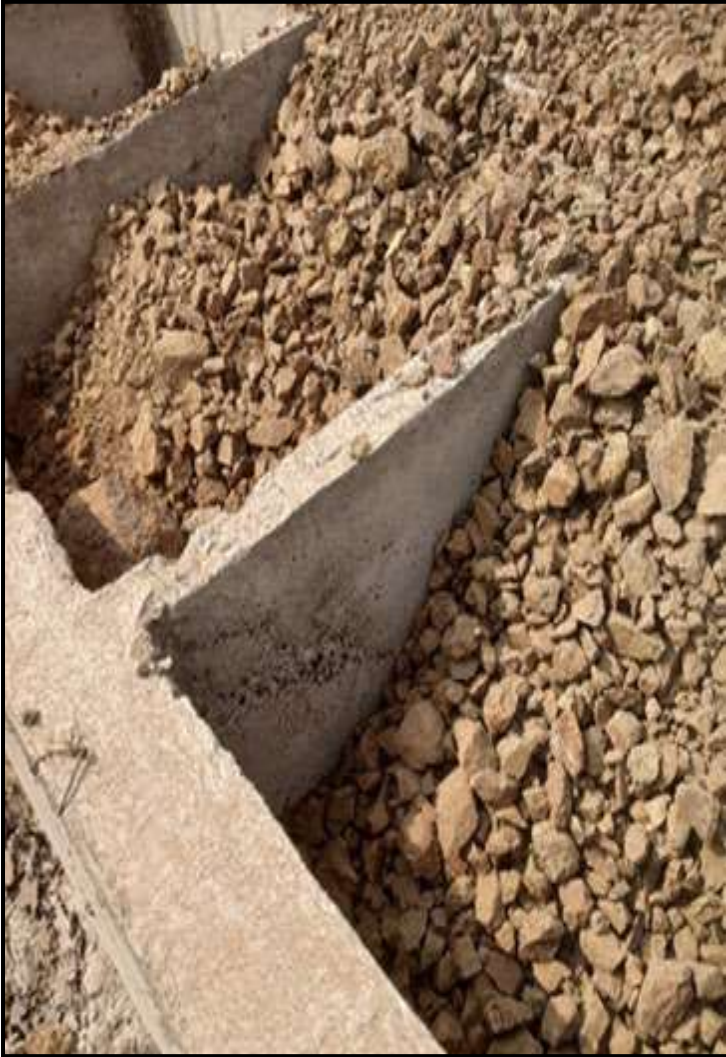
Backfilling in bulk
