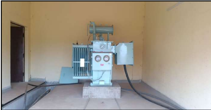
Improper Transformer Cable Connections
