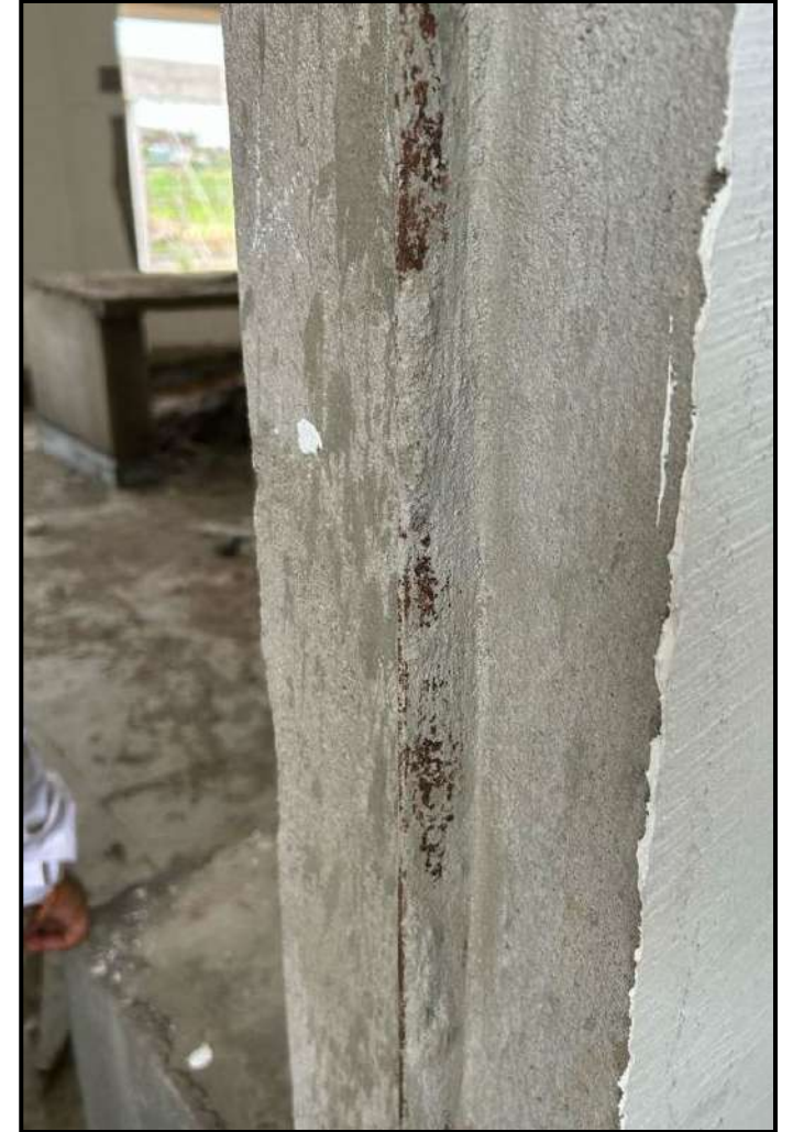
Frame not fitted properly & splashed with mortar
