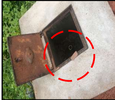
Funnel & Wire Mesh not fixed to Watering Pipe
