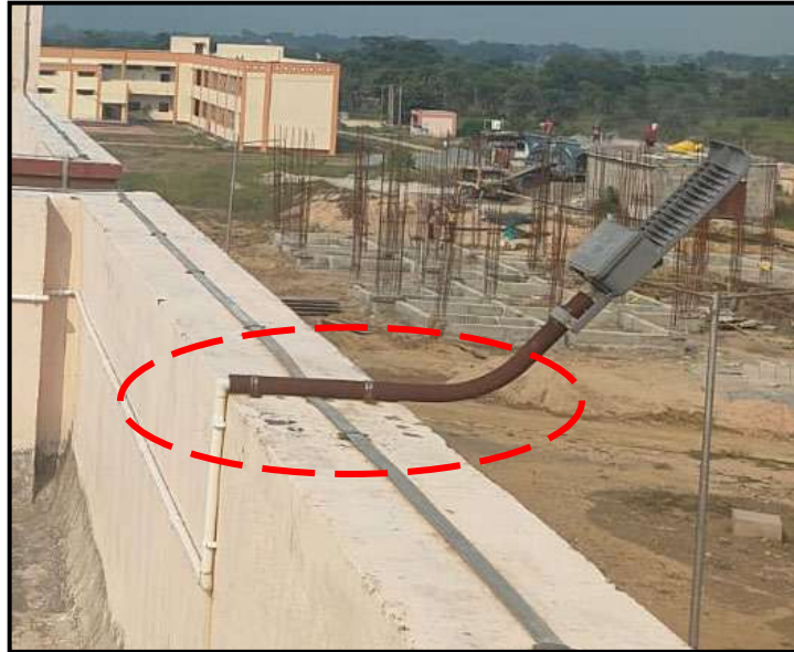
Wrong fixing, No J.Box & Corroded Bracket
