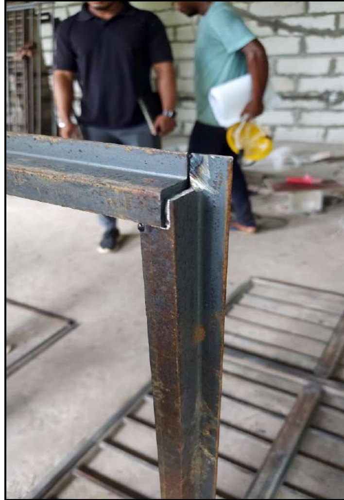
Frame not fitted properly & splashed with mortar
