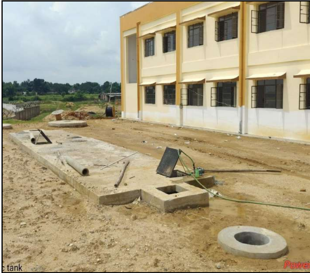
Good work: Inlet/outlet chamber
