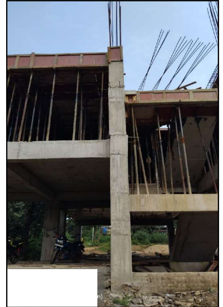
Column not In alignment
