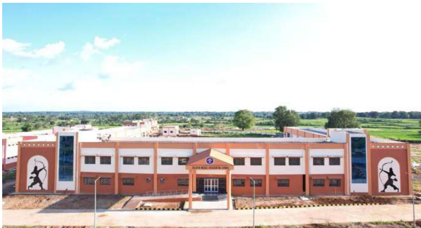
Figure 8.1: EMRS Patthalgaon, Jashpur district, Chhattisgarh
